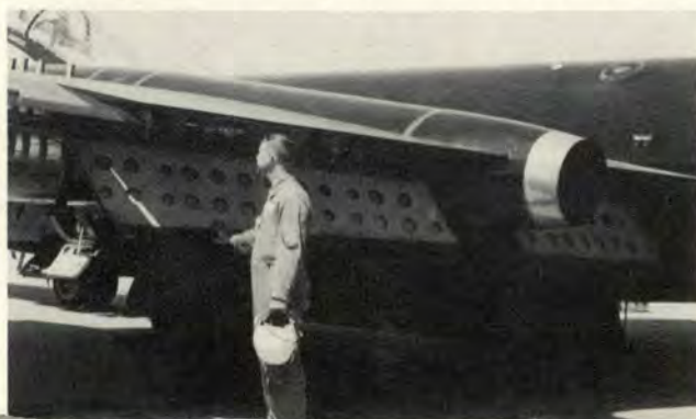
Wing flaps can be used in only two positions: Full Up or Full Down.
