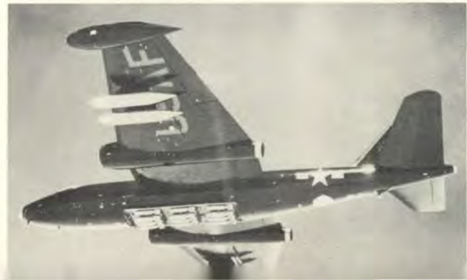
The rotating bomb bay door makes a high speed bombing run possible.
