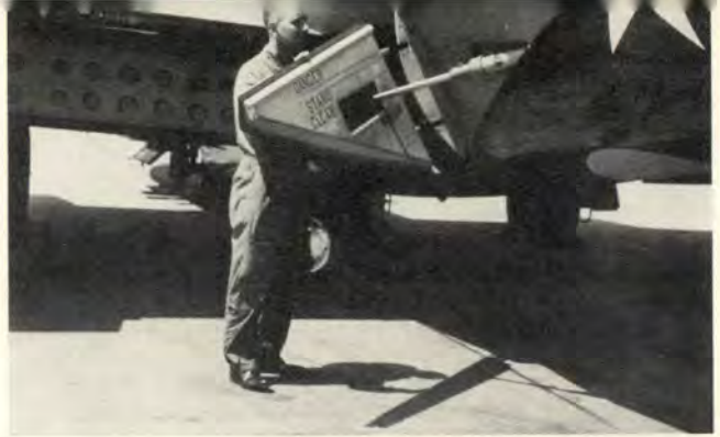
Speed brakes, aptly nicknamed "barn doors," operate hydraulically
